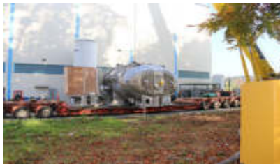
2016 GLAD @ GSI Cave refurbishment
