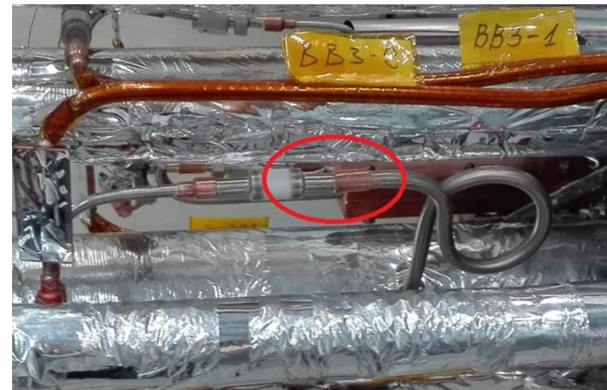
Voltage Breaker view
