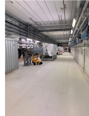
SIS100 Straight 4 Cabling by ELC completed installations
