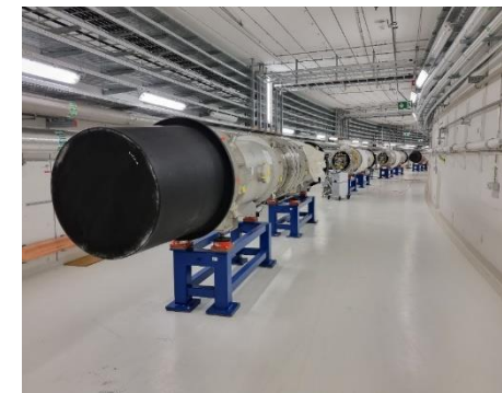
SIS100 Arc 3&2 Dipoles First Phase Mechanical Installation completed
